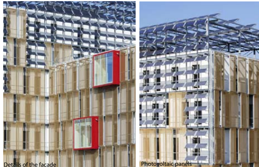
Details of the facade
