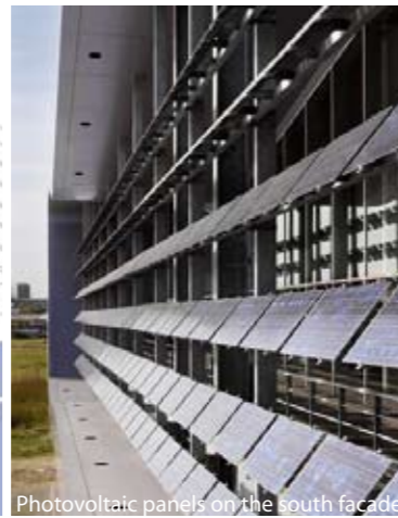
Photovoltaic panels on the south facade
