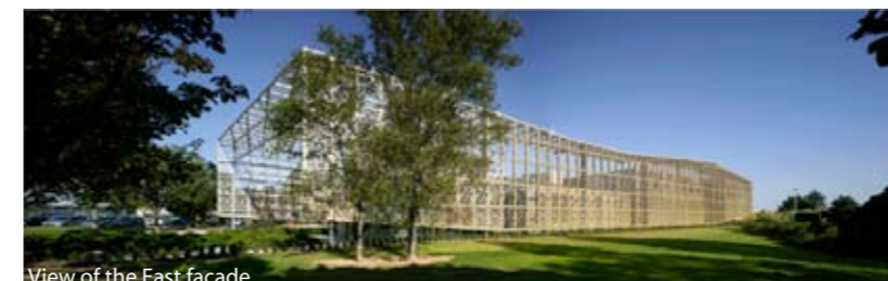
View of the East facade
